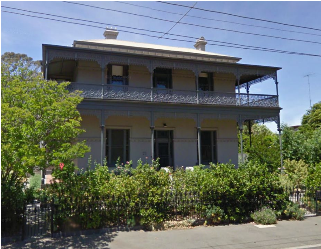
75 Alfred Crescent, North Fitzroy (Google 2012)
